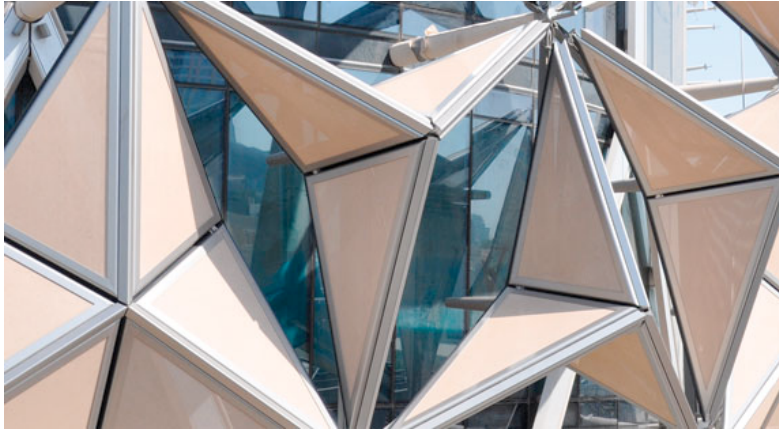
Figure 8. Detail of the shading system components (Council on tall buildings and Urban Habitats, 2013)
