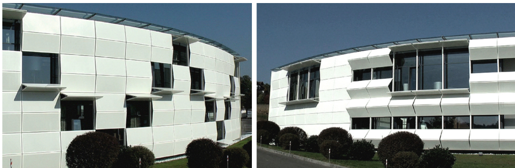
Figure 5. Different positions of the adaptive shading elements on the facade (Archdaily, 2010)
