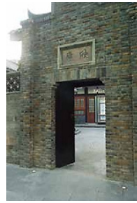
Xin Lu Courtyard :Built in the late Qing Dynasty Function: Ground floor for business with upstairs living
