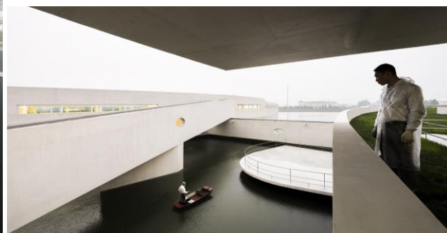
B: looking towards the central court
